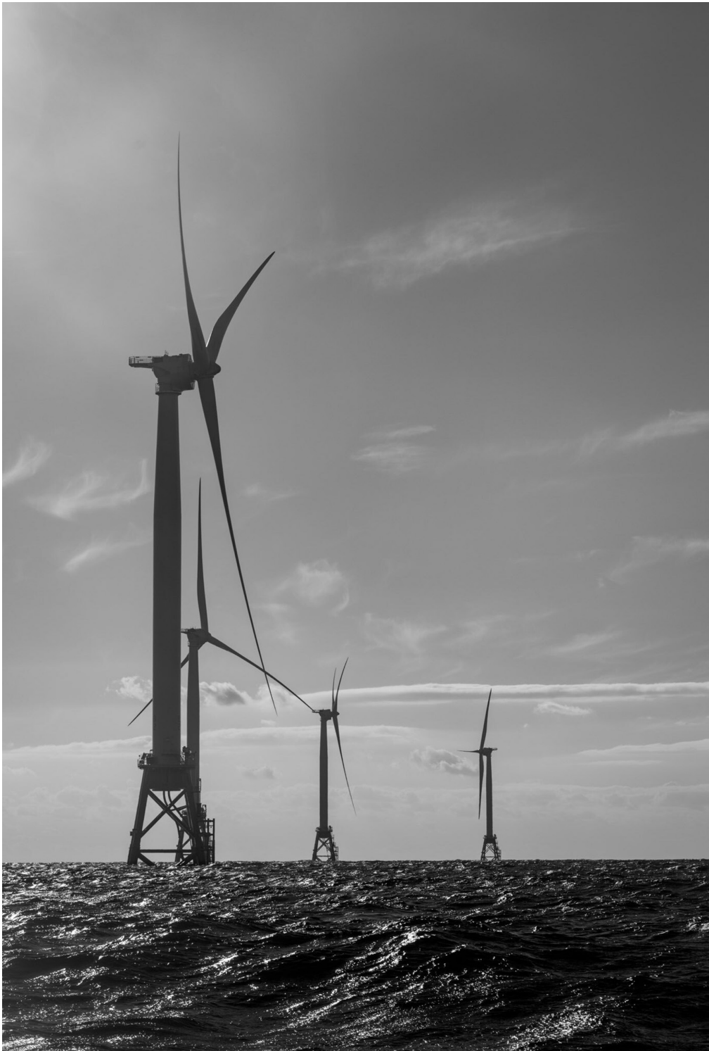
Figure 1. The Block Island Wind Project off the coast of Block Island, Rhode Island, US. Photo courtesy Evan Krape
