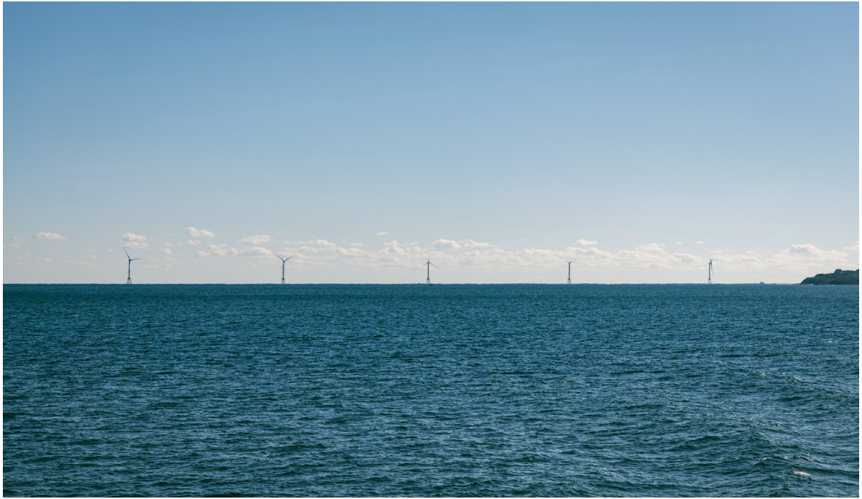
Figure 2. The Block Island Wind Project off the coast of Block Island, Rhode Island, US. A view from the water. Photo courtesy Rafeed Hussain
