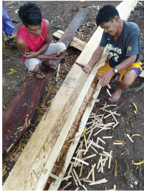
Figure 8. Remelito "Abang" Ilaida, Jr. trims the excess amakan siding , May 2022
