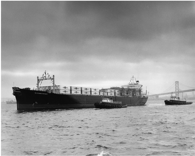
Figure 1. Containership Elizabethport . Originally built as a tanker, the vessel was converted to be one of the early containerships. It is shown here heading into San Francisco in 1962. The new containerships of 2024 have increased their capacity twenty-nine-fold compared with these early vessels. Photograph of Elizabethport , Mystic Seaport Museum, 2024. 66
