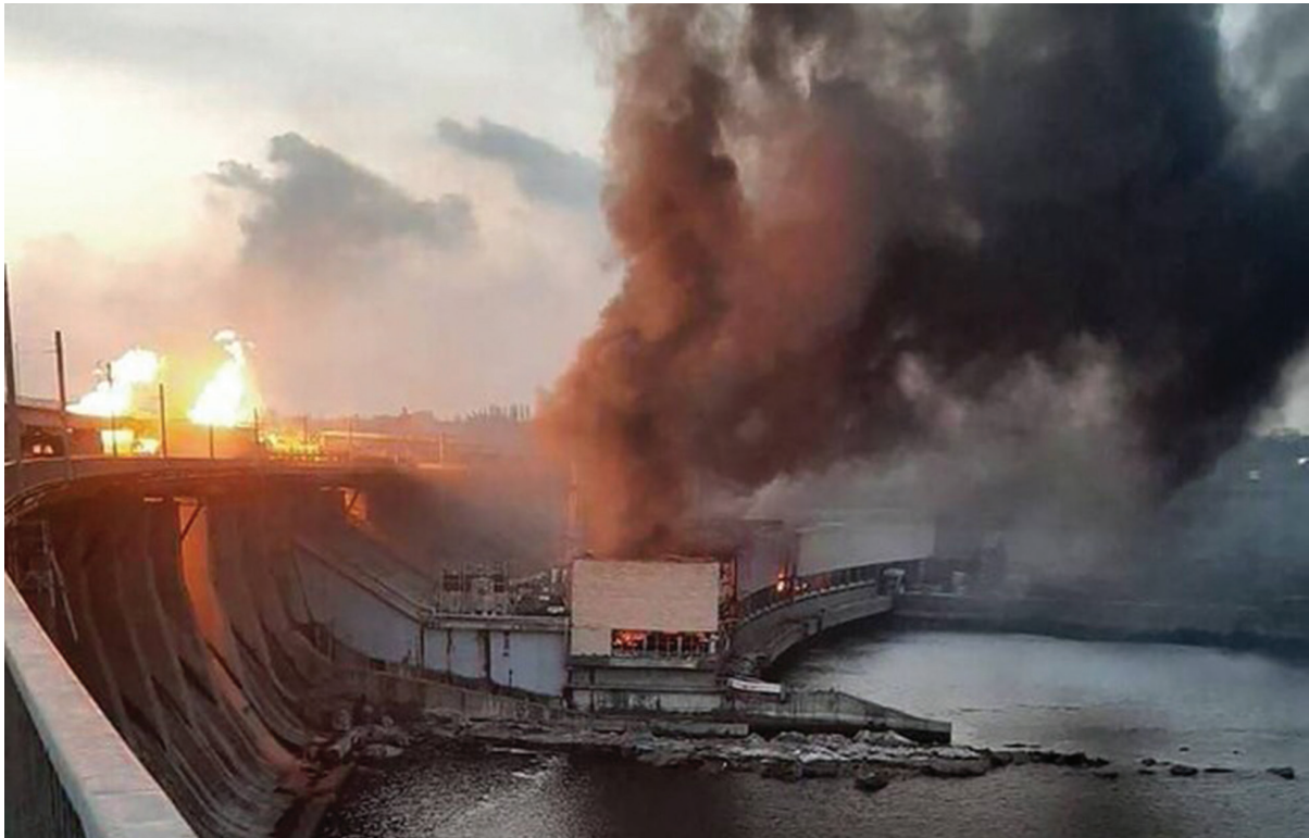
Figure 4. Numerous missile strikes on the Dnipro dam have resulted in a forced water discharge, which previously flowed through the turbines. Photograph courtesy P. Petrenko
